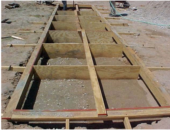
a) Frame Built in a Trench for Long Slab
